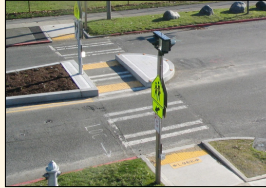
MEDIAN ISLANDS provide a safe place in the middle of the road for people to stop and wait for traffic. If there is a median island, people do not have to wait for traffic to clear in both directions. They can cross when traffic is clear in only one direction.
